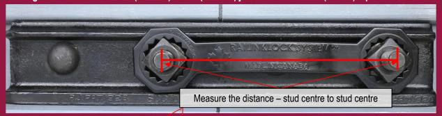
12-inch - designed to be used with 25" (635 mm) or 36" (914 mm) joint bars with 1 5/8" (41 mm) square nuts and 24" (610 mm) or 36" (914 mm) joint bars with 1 3/4" (44.5 mm) square nuts.
